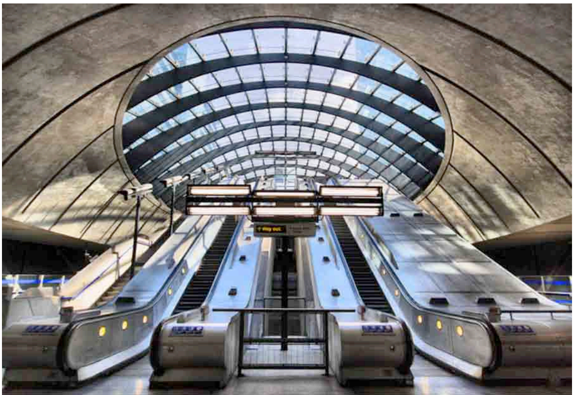
参考事例：Canary Wharf Station (London)
