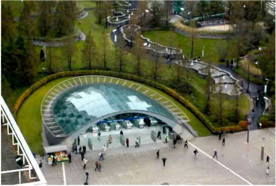
参考事例：Canary Wharf Station (London)
