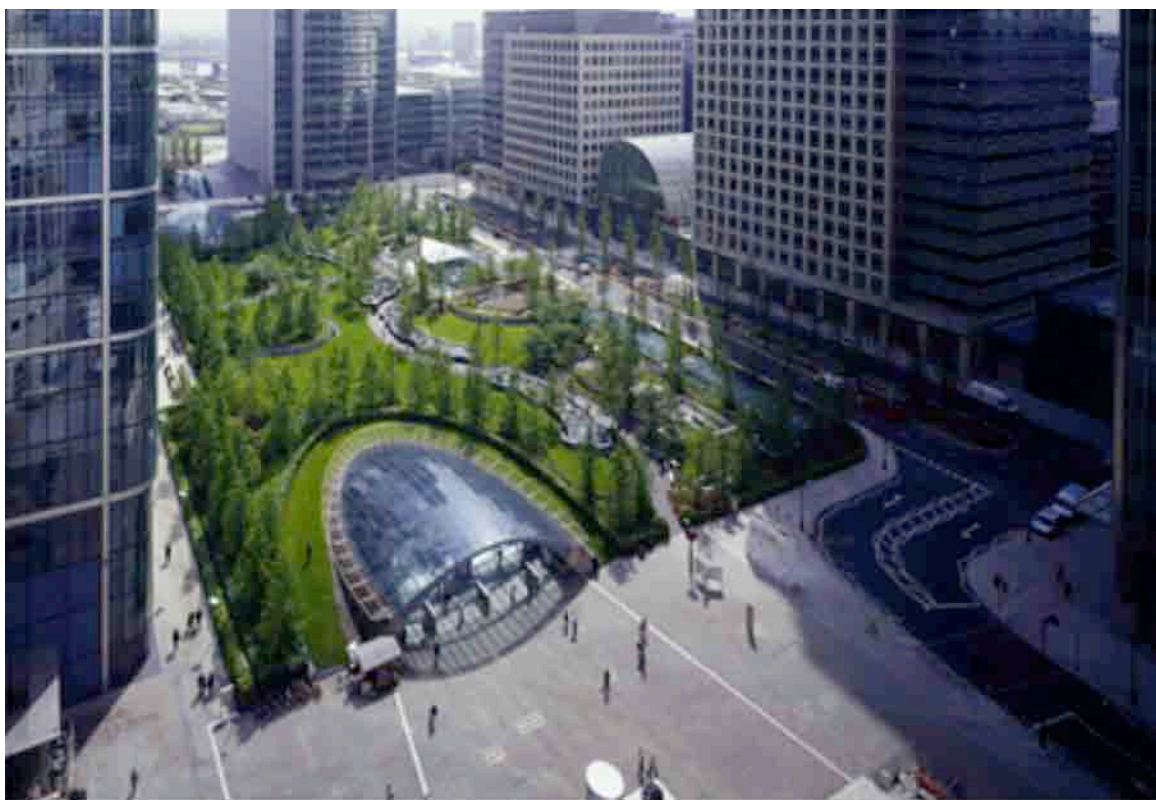
参考事例：Canary Wharf Station (London)
